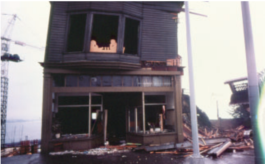
2001 First Avenue studio during demolition, 1978
